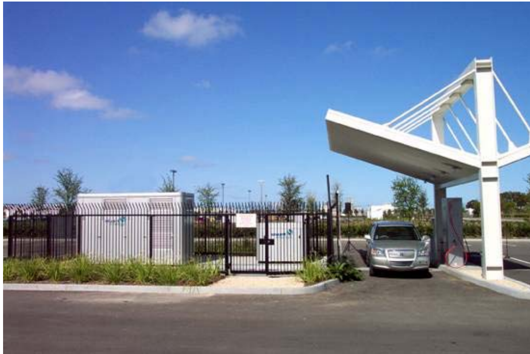
Figure 14 - Hydrogen Fueling Station based on Electrolysis (courtesy of Stuart Energy Systems)
